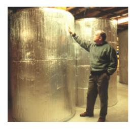
The supply feed to the collector array is piped from one tank while the hot water return from the collectors flows into the other tank. Since both tanks develop stratification, the coolest water is delivered to the array which enhances the collection efficiency. Radiant heat distribution delivers the solar heat throughout the house.
