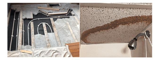
So it was necessary to rip the flooring up and chip through the concrete to expose the tubing to find the leak. Alas, there was no leak in the floor. One of the workmen discovered stained ceiling tiles in the basement and the source was discovered to be a first floor manifold that
