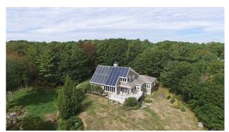
We're sliding toward the really cold months with snow and ice storms the norm. The best thing a properly sited solar house has going for it in the fall and winter is the sun angles - shinning at a much lower angle into our south-facing home. That generates considerable passive solar heat. Our front room can approach 80 degrees even on the coldest of days, thus the need to disipate the extra warmth by opening several windows.
